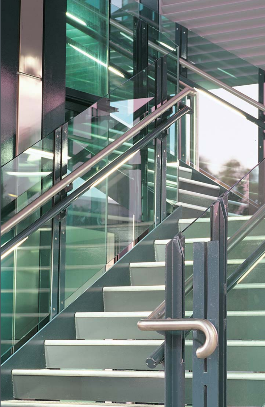
Busways Transit Station
